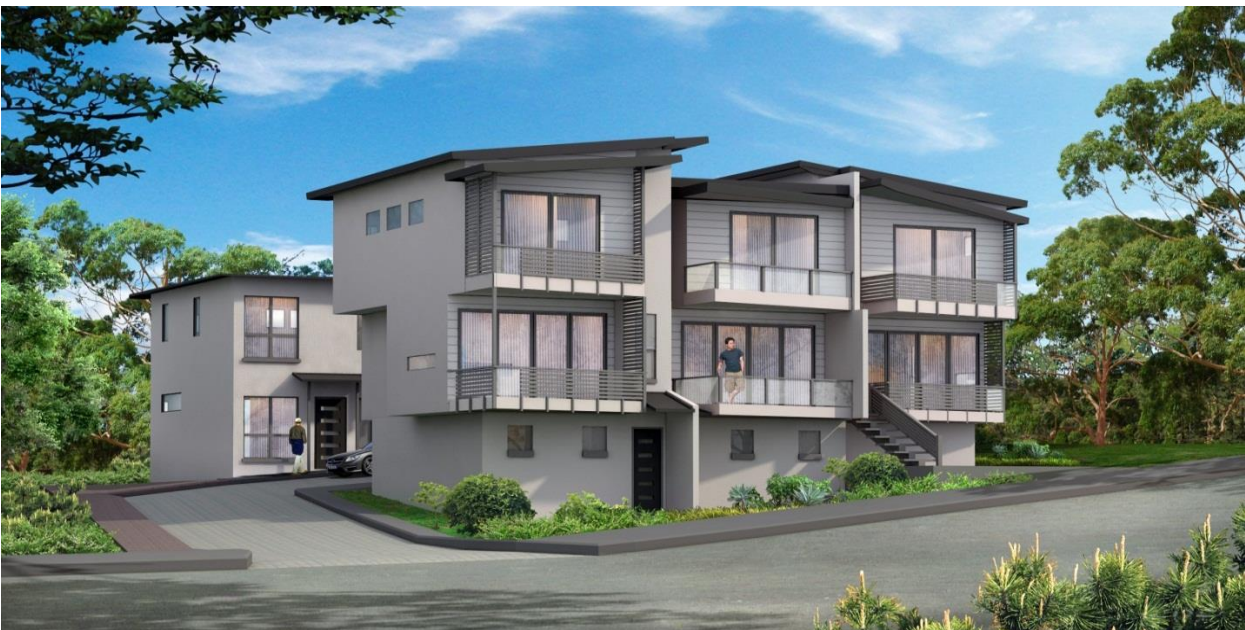
15 Rutland Street Coorparoo Qld - construction of 5 townhouses
